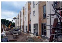
Following a lengthy and very competitive tender process, Deeside Timberframe Ltd were appointed by Main Contractor, Russells Construction, to design, supply and install the timber frame structures for the residential part of this large scale project.
